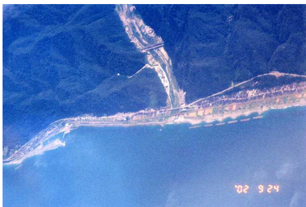
Photo 1. Example of beach erosion by decrease in sediment supply from a river
