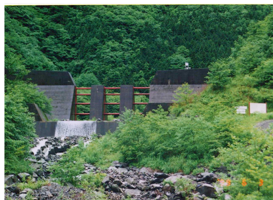
Photo 2. Example of sabo dam which controls the size of debris and stones
