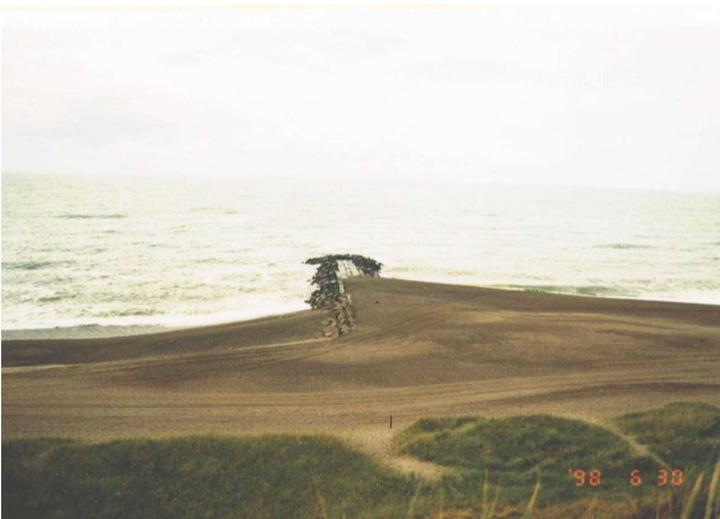
Photo. 3 Longshore sediment transport around a groin
